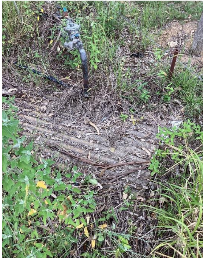
Image 5: Example of fibrous corrugated sheets observed near the Site entrance and adjacent to the mains water valve (taken on 25/01/2024)
