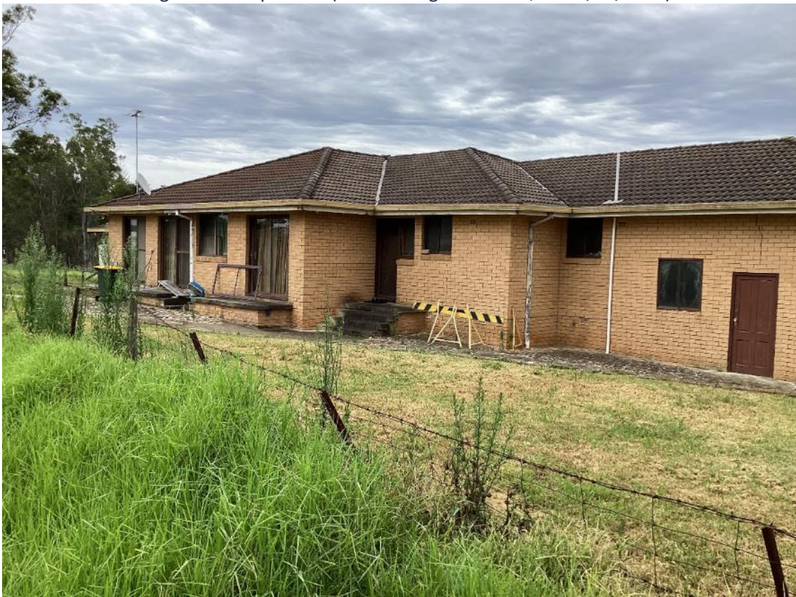
Image 34: Residence in western portion of Lot B (taken facing west, on 25/01/2024)
