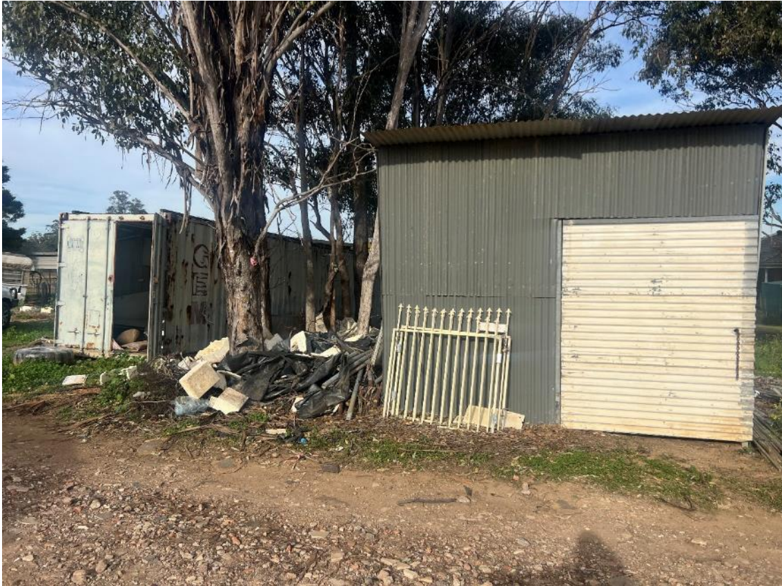
Image 11: Shipping Container 1 and Storage Shed (taken facing south-east, on 24/07/2024)
