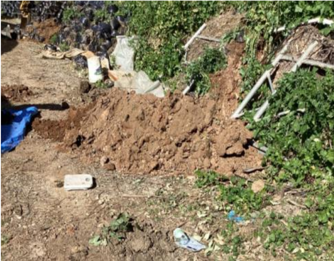
Image 28: Stockpile SP3 (dam wall, adjacent to Dam A) in Lot A DP411211 (taken facing north, on 24/07/2024)
