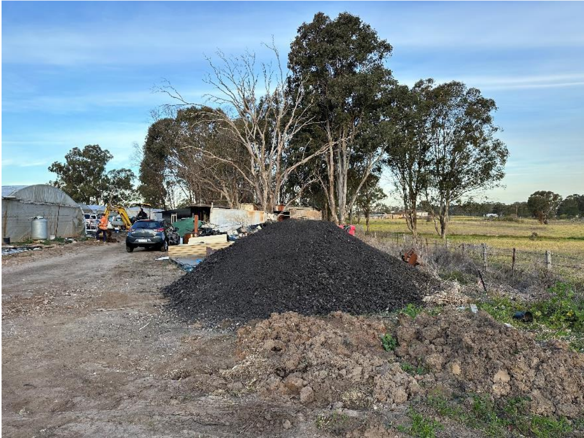
Image 33: Stockpile SP1 (taken facing south east, on 24/07/2024)
