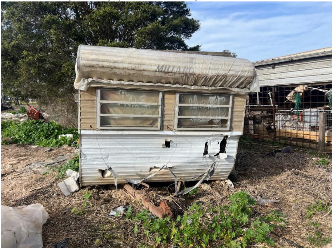
Image 10: Dilapidated caravan (taken facing south east, on 24/07/2024)
