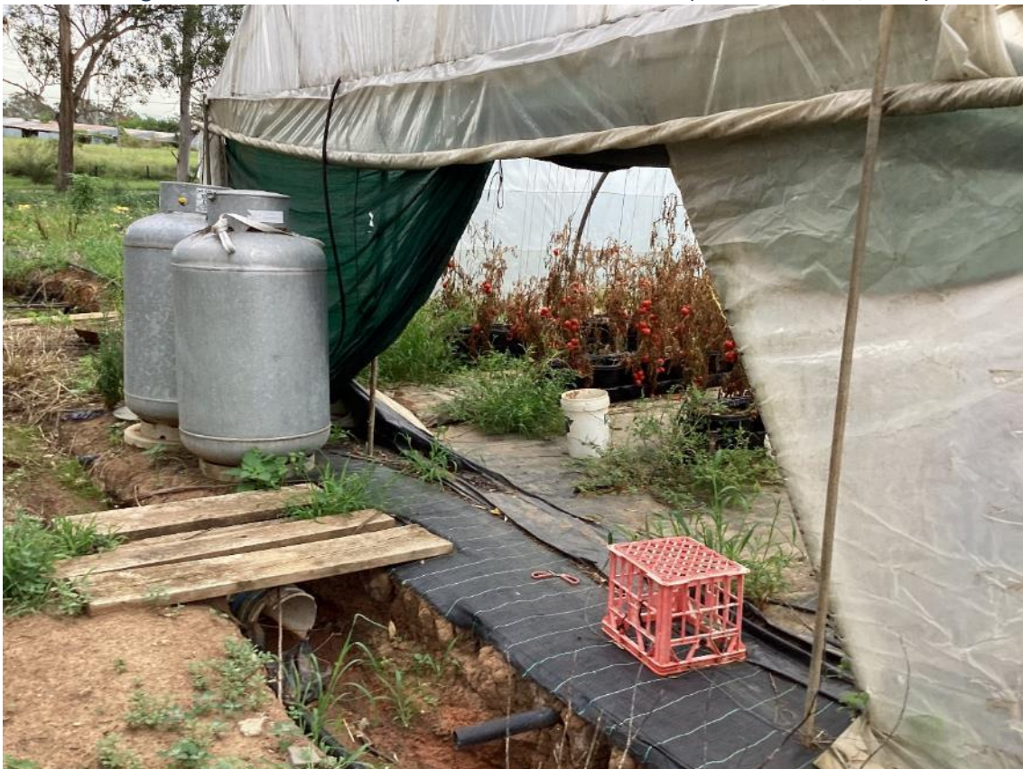
Image 8: Example of liquified petroleum gas tanks adjacent greenhouses and drainage line running adjacent greenhouses in Lot A DP411211 (taken facing north-west on 25/01/2024)
