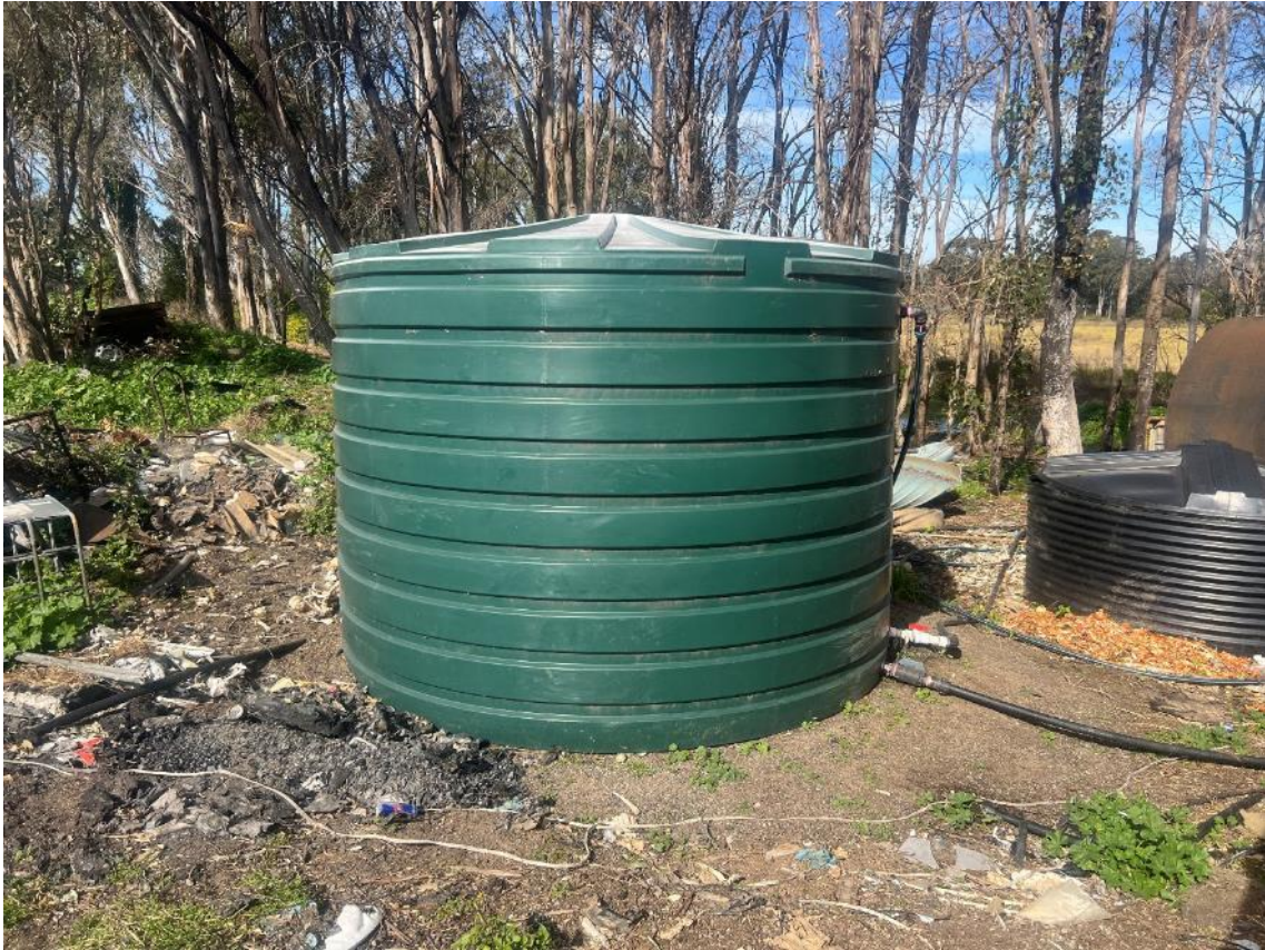
Image 29: Tank A (taken facing south, on 24/07/2024)
