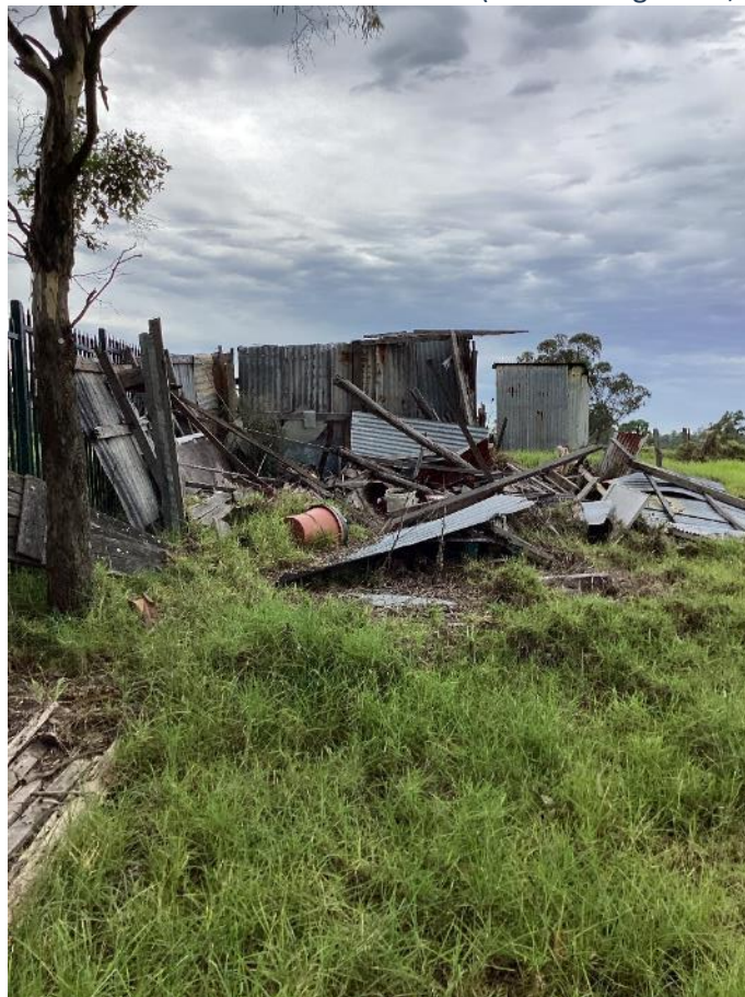
Image 40: Example of remnant and demolished corrugated metal sheds and associated debris within the central northern portion of Lot B DP411211 (taken facing east, on 25/01/2025)
