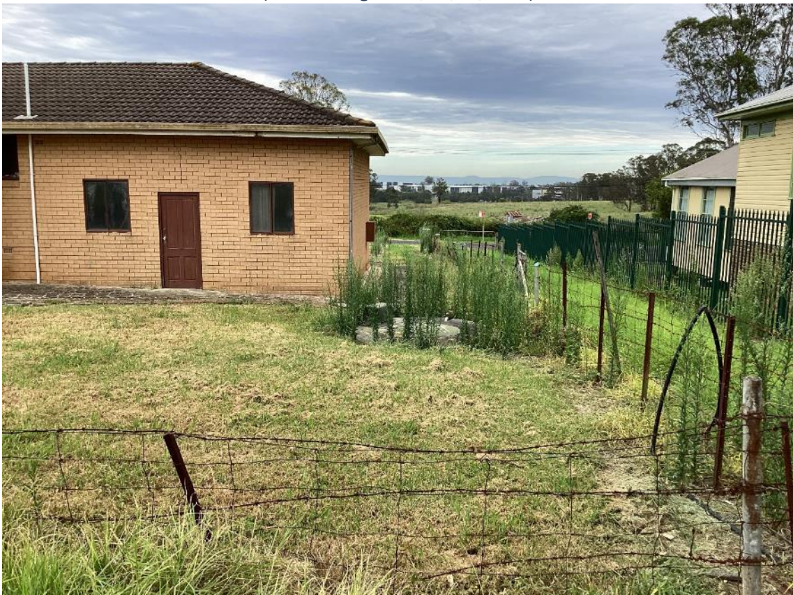
Image 38: Lot B DP411211 Residence septic tank located in the backyard within fenced area (taken facing west, on 25/01/2025)
