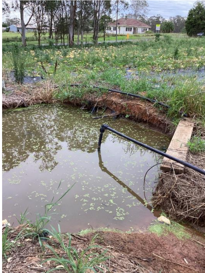
Image 7: Dam B south-east portion of Lot A DP411211 (taken on 25/01/2024)
