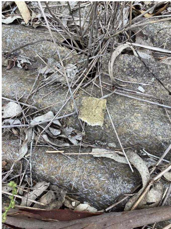
Image 6: Example of fibrous corrugated sheets observed near the Site entrance and adjacent to the mains water valve (taken on 25/01/2024)
