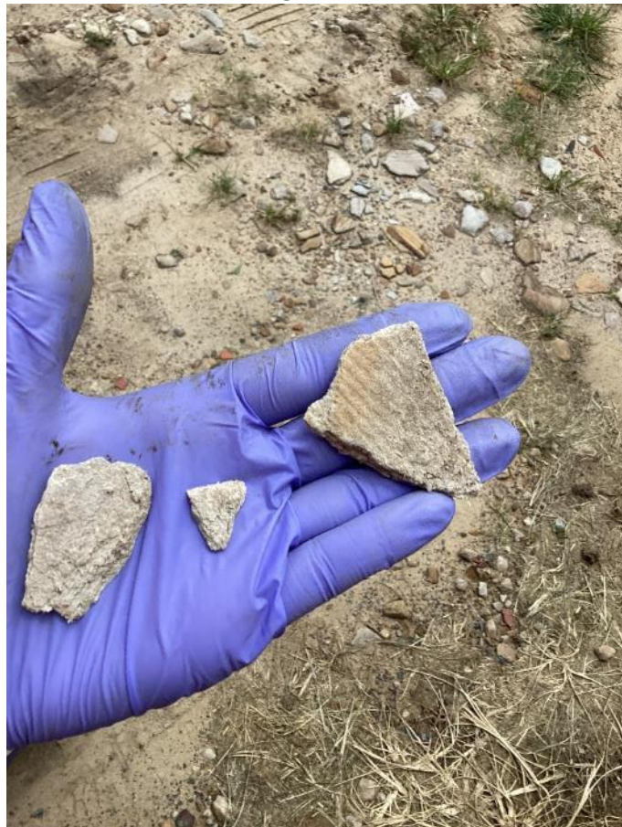
Image 50: Representative fibre cement fragments taken adjacent STP12 (taken on 07/02/2024)
